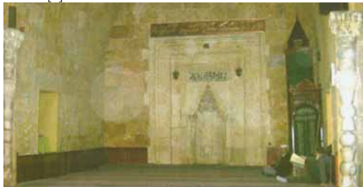
Figure 6: One of the columns shown on the right
