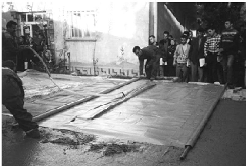
Figure 2. Application of vacuum process.
