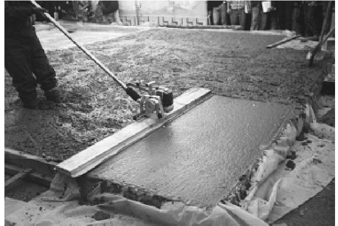
Figure 1. Compaction of concrete with vibrating screed
