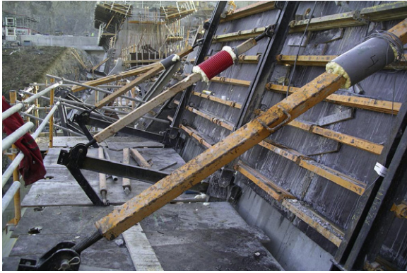
Fig. 5. Instrumented trusses placed at the construction site.
