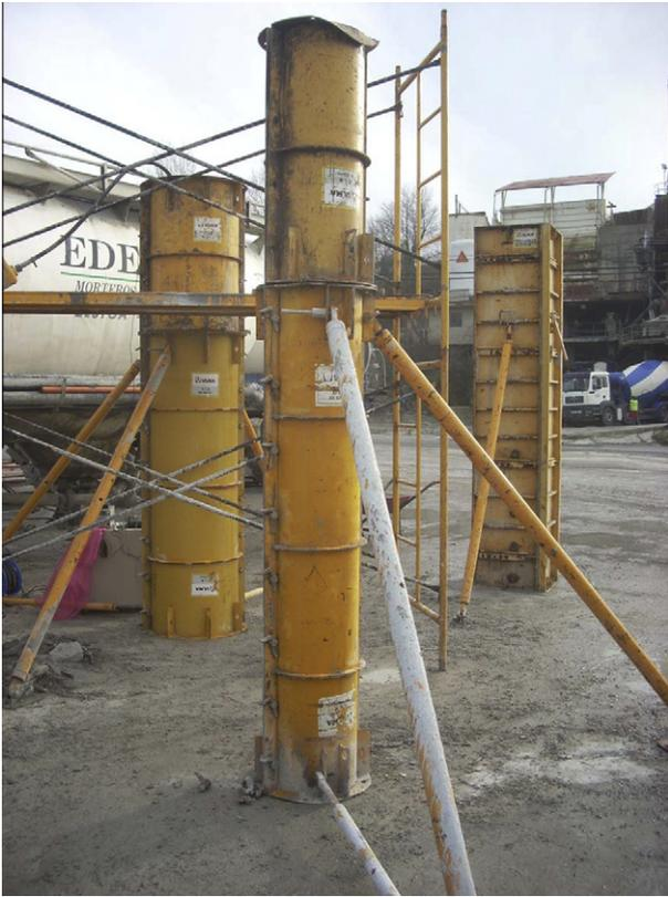
Fig. 3. Formworks placed at construction site.
